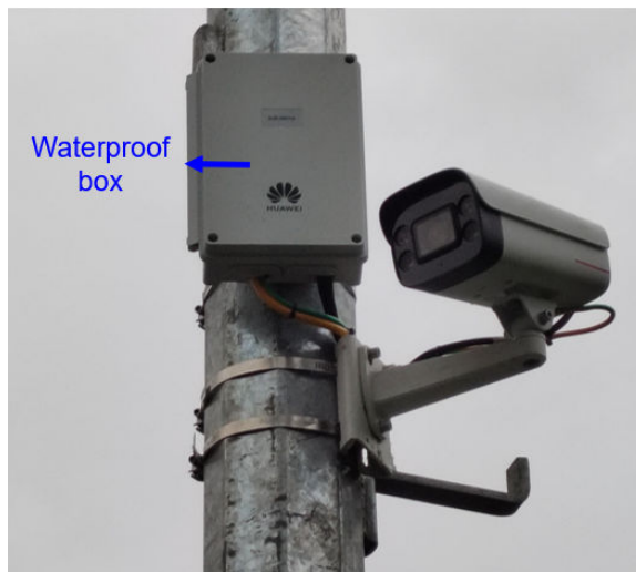
Figure 6-10 Waterproof box installation illustration
